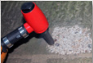
Reducing Levels on Concrete
