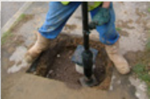
Reinstatement Compaction
