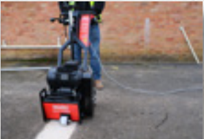
Roughening Concrete
