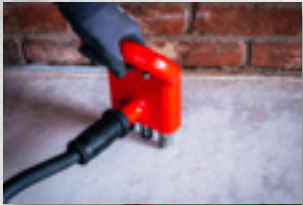
Reducing Levels on Concrete
