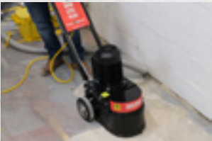
Grinding Concrete
