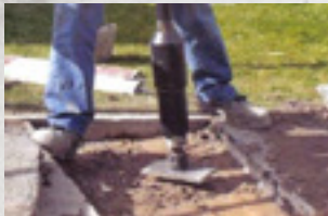
Back Fill Compaction
