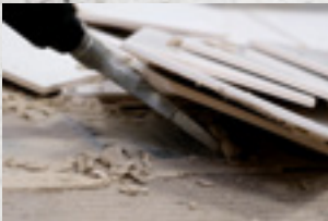
Ceramic Tile Removal
