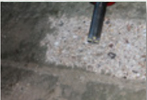
Roughening Concrete
