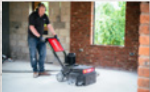
Grinding Concrete
