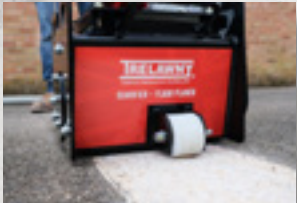
Reducing Levels on Concrete
