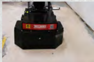
Polishing Concrete Floors
