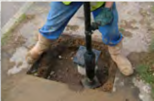
Reinstatement Compaction
