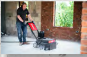
Grinding Concrete
