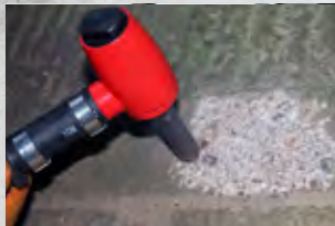
Reducing Levels on Concrete
