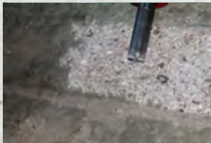
Roughening Concrete
