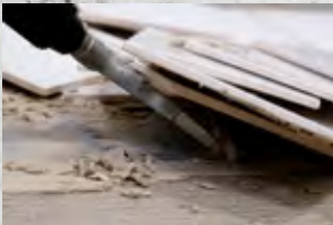
Ceramic Tile Removal
