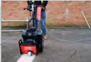
Roughening Concrete
