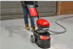
Grinding Concrete
