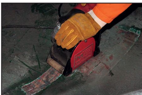
HAZARDOUS PAINT REMOVAL
