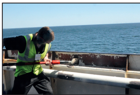
CLEANING STEELWORK
