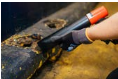
CLEANING STEEL STRUCTURES
