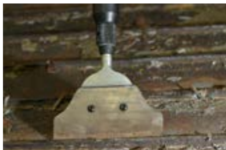
SHIP DECK RUST REMOVAL
