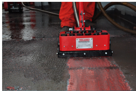
REMOVAL OF ANTI-SKID COATINGS
