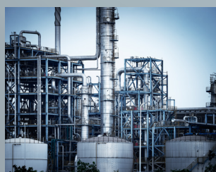
CHEMICAL PROCESSING PLANTS
