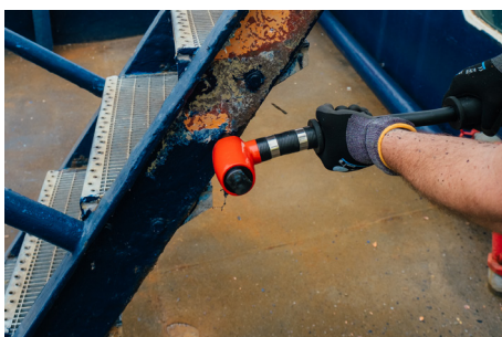
CORROSION REMOVAL
