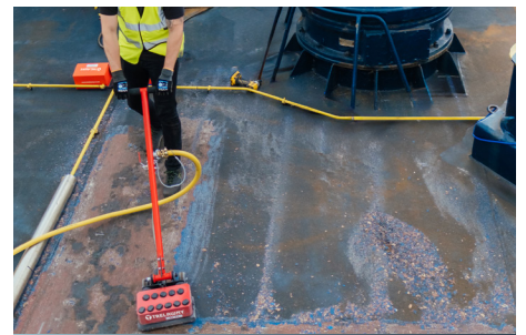
DUST FREE DESCALING
