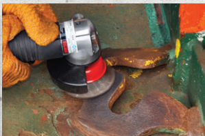
Weld Seam Removal
