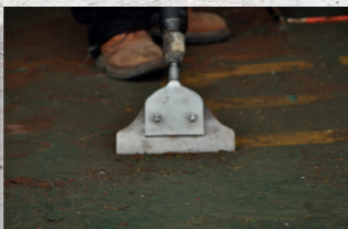
Ship Deck Rust Removal
