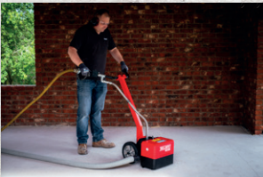
Fast Removal of Concrete
