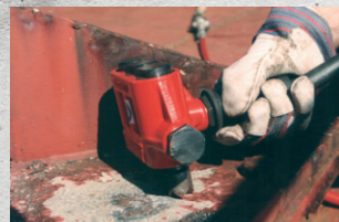
Thick Paint Removal
