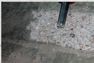
Roughening Concrete
