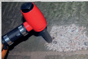
Reducing Levels on Concrete
