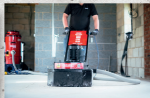
Removing High Spots
