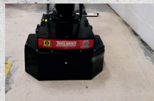
Polishing Concrete Floors
