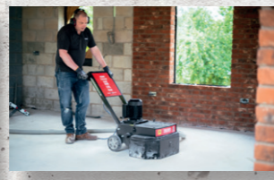
Grinding Concrete
