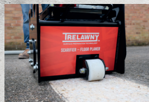
Reducing Levels on Concrete
