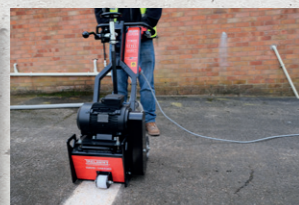
Roughening Concrete
