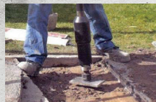
Back Fill Compaction
