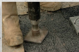
Asphalt Compaction
