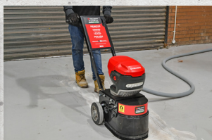
Grinding Concrete
